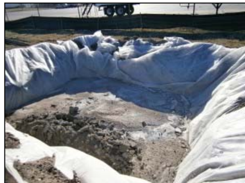
Plate 3.2 Concrete washout area
