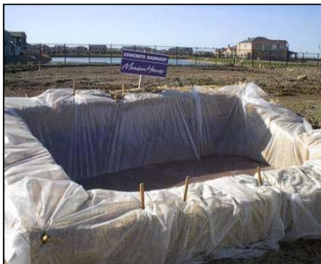
Plate 3.1 Concrete washout area
